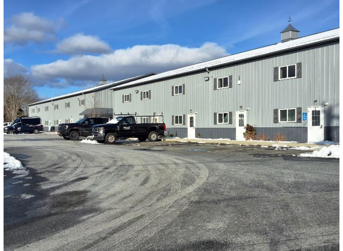
New Contractor Bays - Osterville
