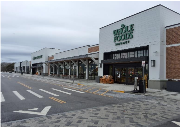
Home Depot renovation and expansion
