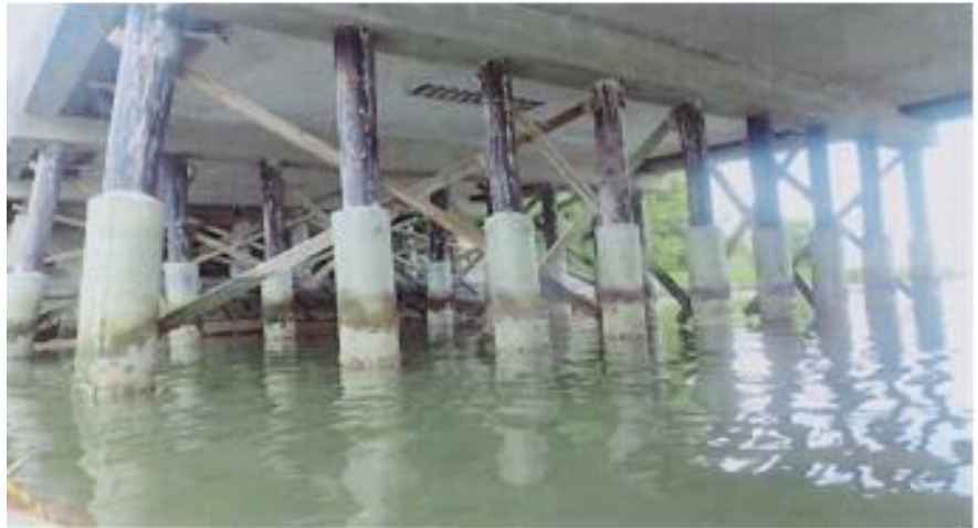
Bumps River Bridge
