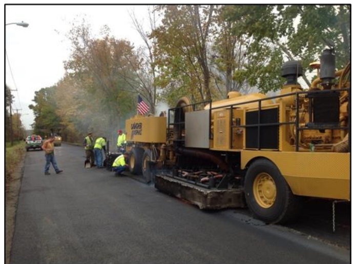
Sunderland Road – Hot In Place Process
