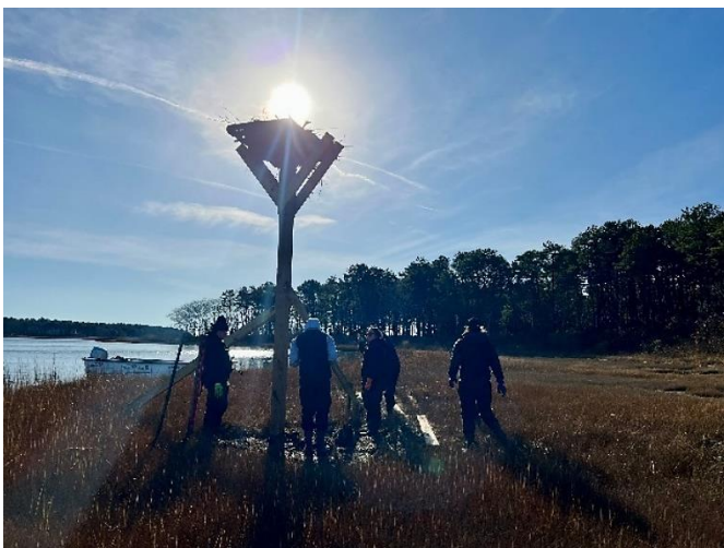
Home for the Holidays! December osprey pole installation in Pinquicket Cove.
