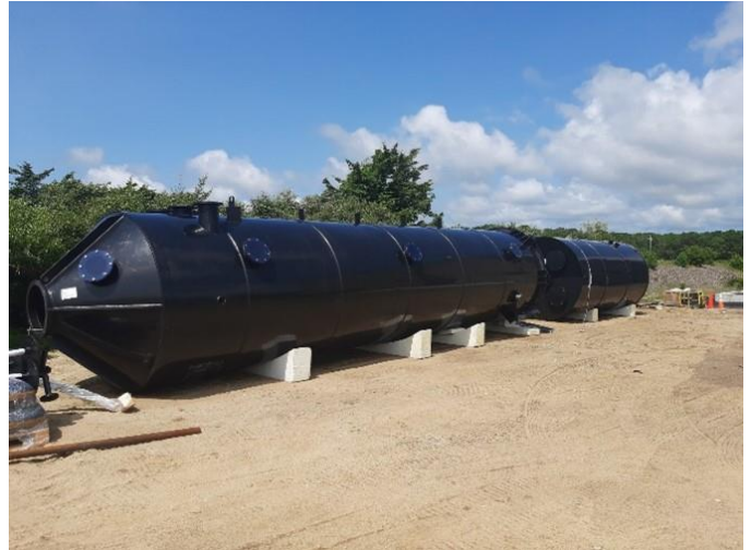
New Odor Control Vessels Installed for Solids Handling Project
