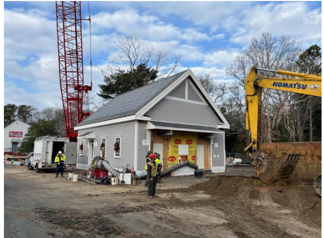
Phinney’s Lane Pump Station Project
