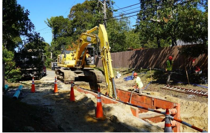
Strawberry Hill Road Sewer Expansion Project
