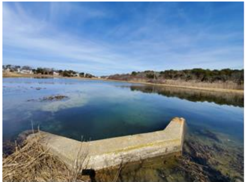
Hawes Ave -Culvert Reconstruction
