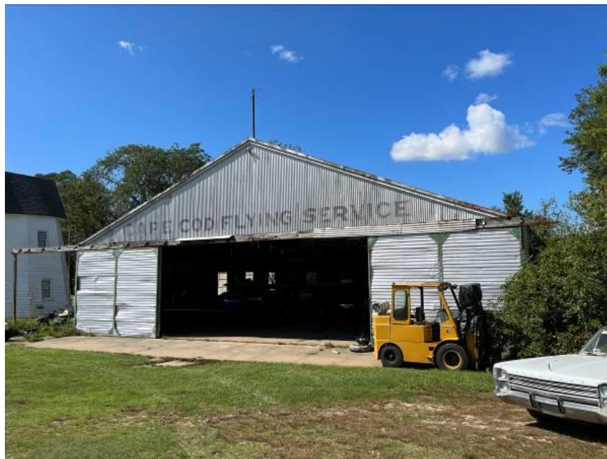
Cape Cod Airfield -Hanger Repair
