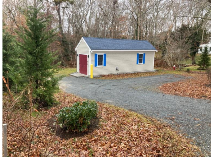
The new permanent interconnection with the COMM water system on Longview Drive in Hyannis
