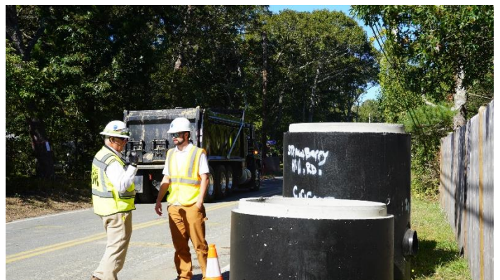
Sewer construction on Strawberry Hill Road
