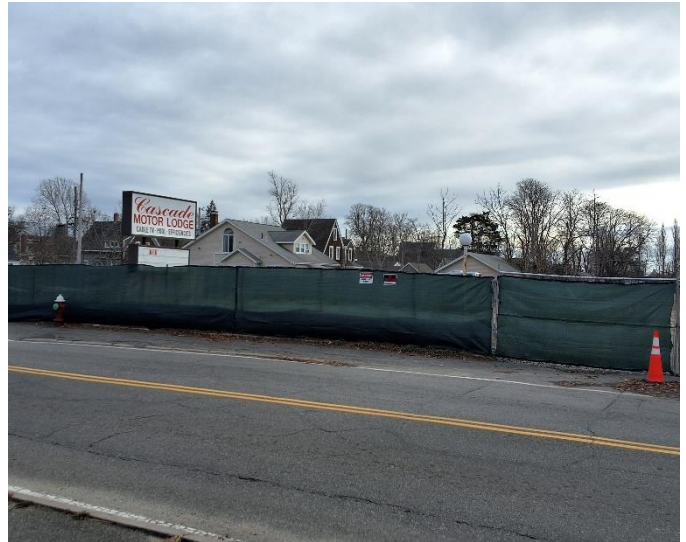
Cascade Demolition - Hyannis
